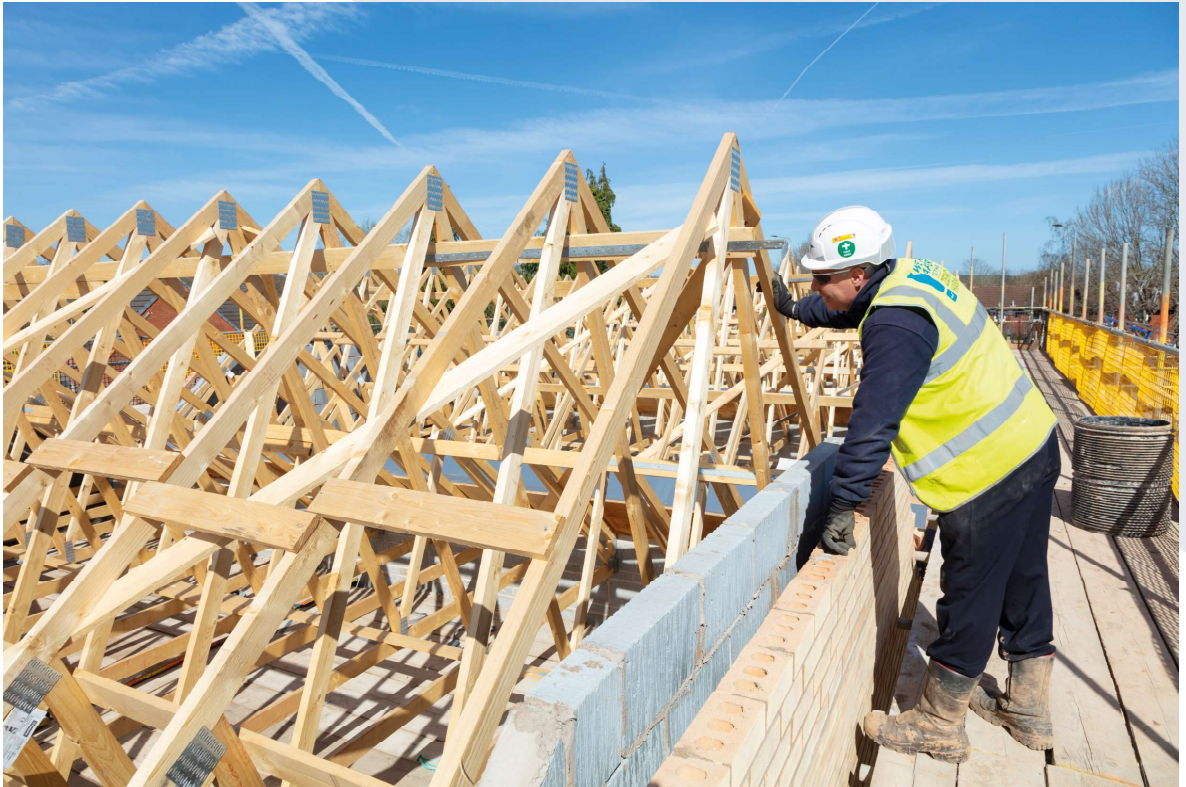
Engineer inspecting the roofs at Willowbrook West, St Mellons
