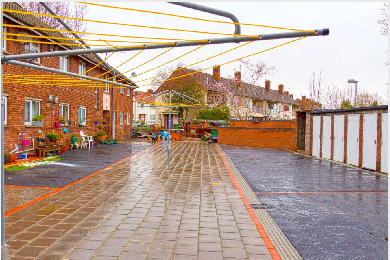
Courtyard improvements in Morris Avenue
